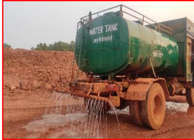
Water sprinkling through tanker.
