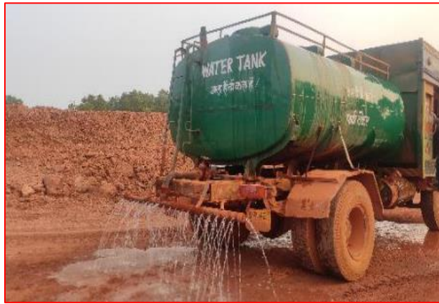
Water sprinkling through tanker.
