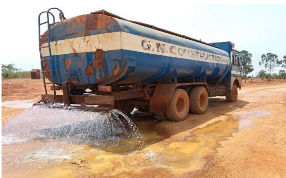
Water Sprinkling in haul road
