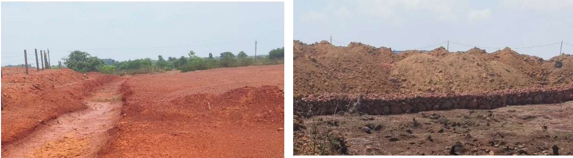
Photographs of garland drains and parapet wall
