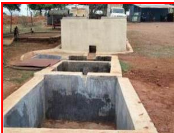
Washing Ramp with Oil & Grease Trap
