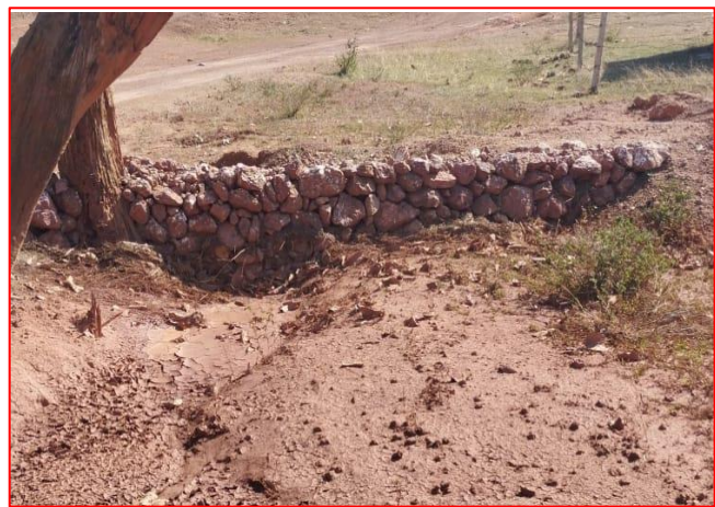
De-siltation Arrangement
