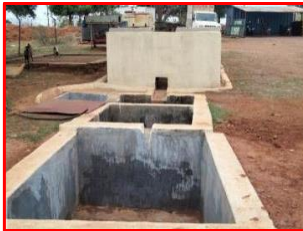
Washing Ramp and Oil and Grease Trap
