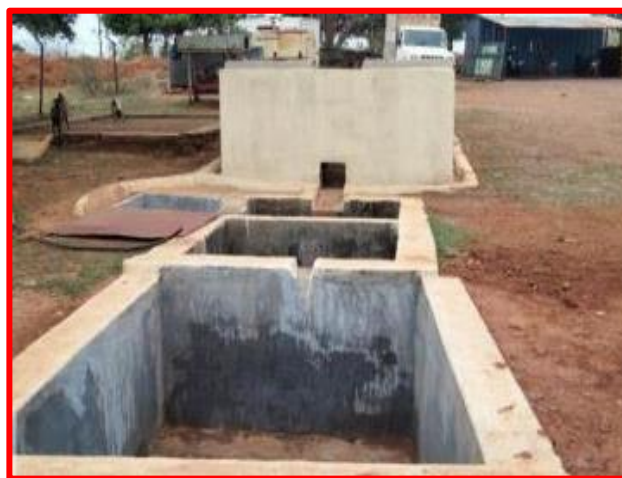
Washing Ramp and Oil and Grease Trap
