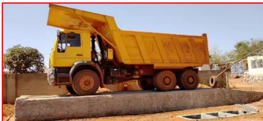
Washing ramp with Oil and Grease Trap
