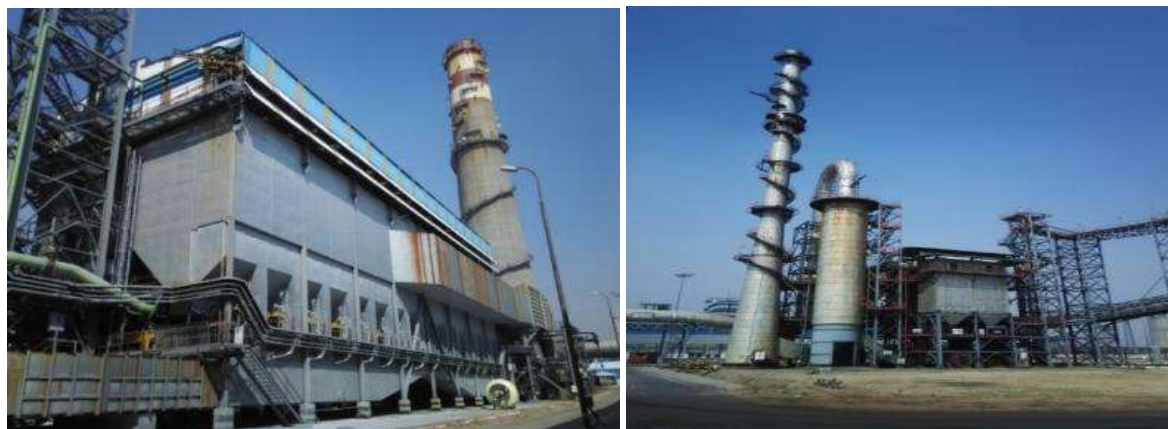
Photo No 5 – Dry Scrubbing System for Pot Room and Anode baking System respectively.
