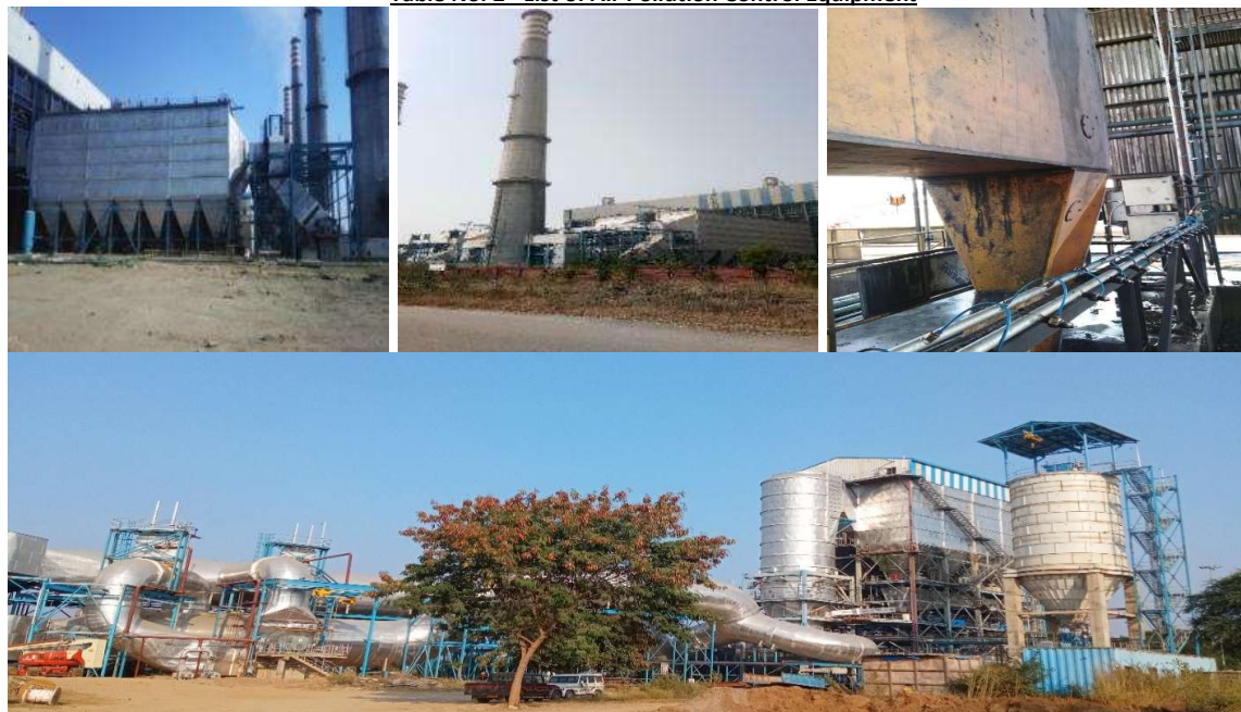
Photo 1 – ESP along with Stack and Dust Suppression System in CPP respectively along with new commissioning of FGD
