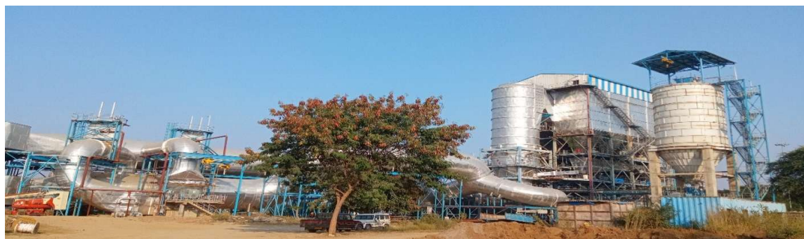
Photo 1 – ESP along with Stack and Dust Suppression System in CPP respectively along with new commissioning of FGD
