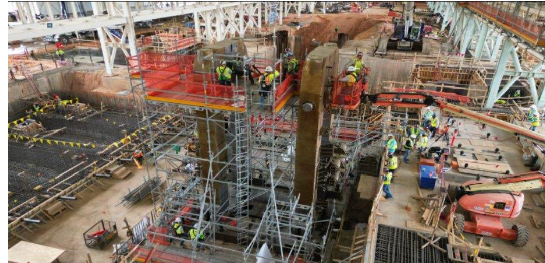
Hot finishing mill stand installation
