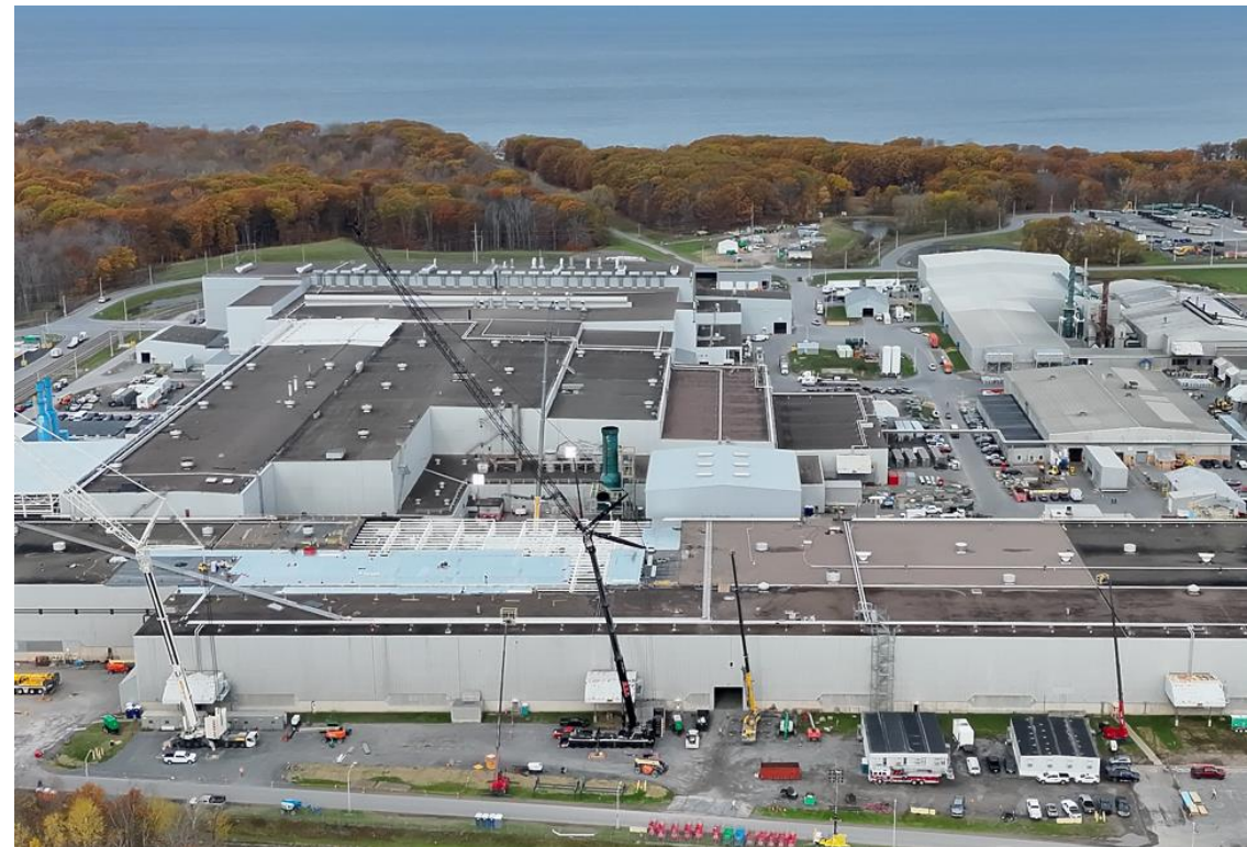
Roof repair progress
