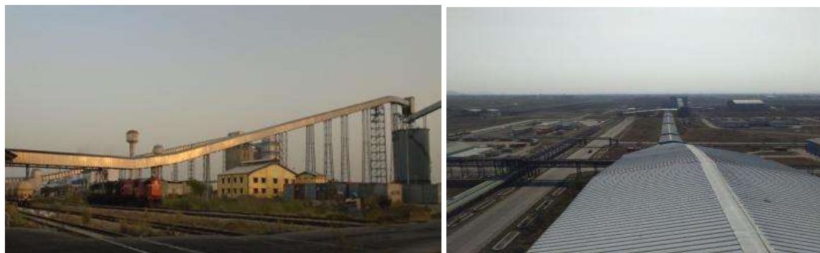
Photo 4 - Conveyer belt For Alumina & Pet Coke Handling and Coal respectively
