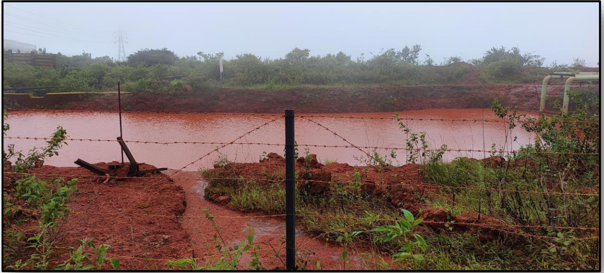
PHOTO 3: Showing Settling Ponds
