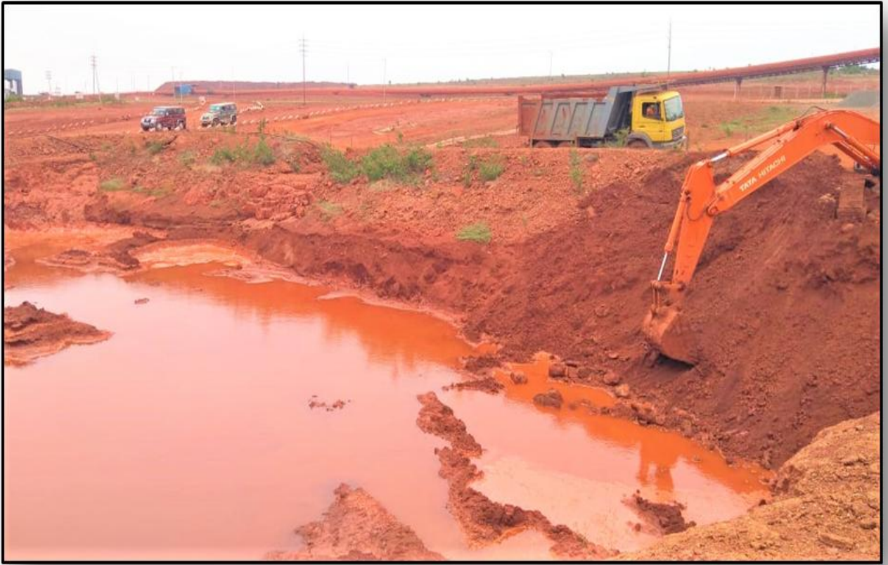
PHOTO 4: Showing Settling Pond Desilting
