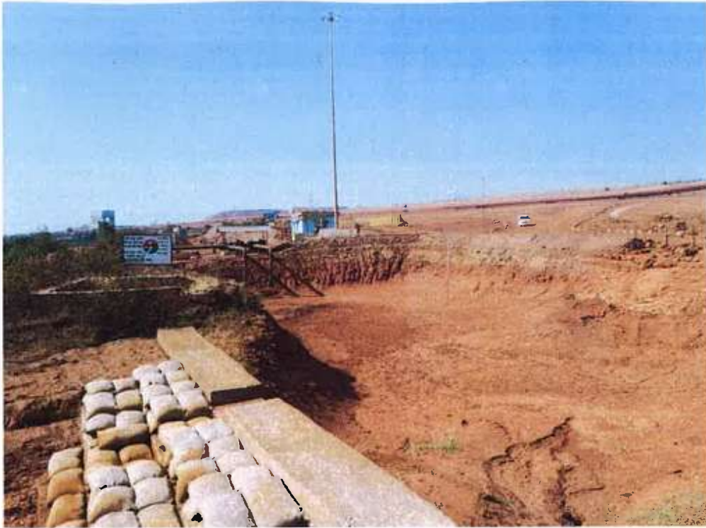
Figure 2: View of the reconstructed settling pit near the mine entrance
