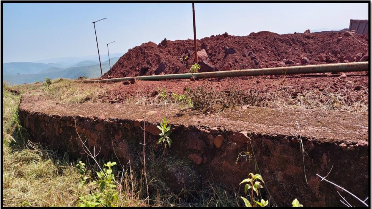
PHOTO 3: Showing Settling Ponds
