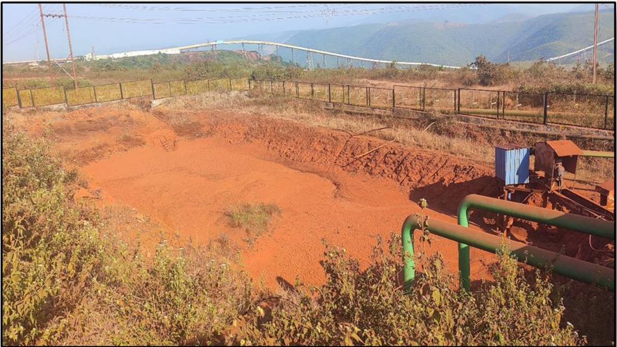
Settling Pit Near Crusher House
