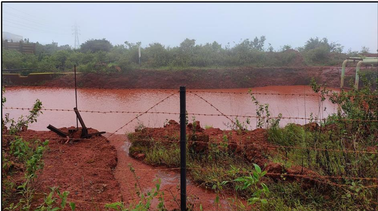
Settling Pond-2 Near Mines Entrance
