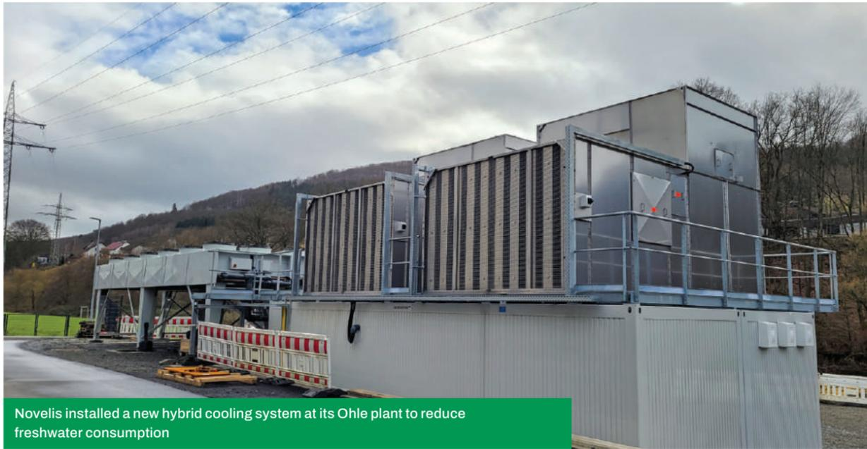
Novelis installed a new hybrid cooling system at its Ohle plant to reduce freshwater consumption
