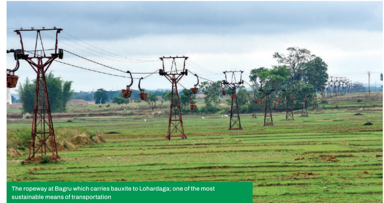
The ropeway at Bagru which carries bauxite to Lohardaga; one of the most sustainable means of transportation
