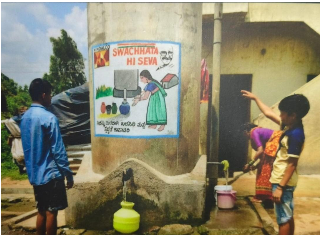
Figure 3: Community water tap structure observed in Belagavi
