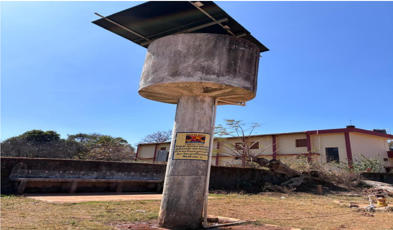
Figure 2: Solar light installed as part of Solar energy support intervention in Lohardaga
