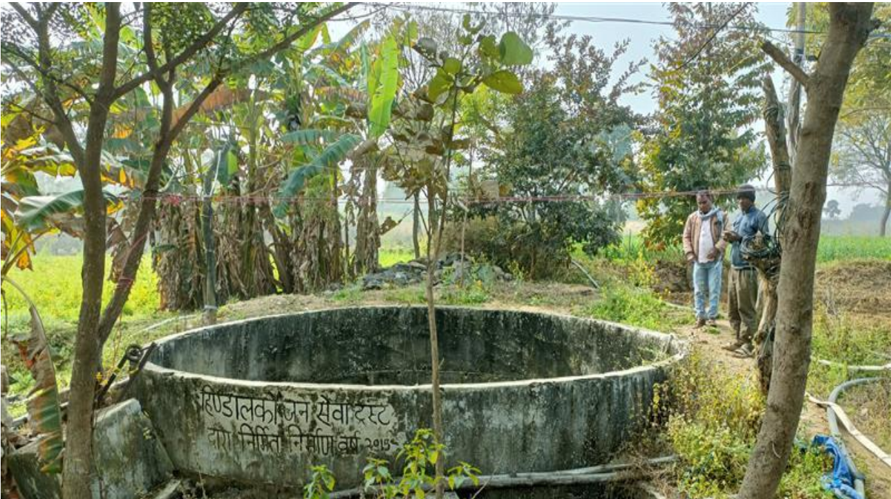
Figure 1: Improved groundwater recharge activity done as part of water conservation and harvesting intervention in Renukoot
