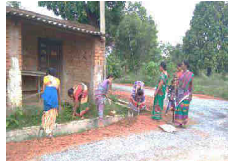
Drain Cleaning by SHG women at Pondoloi
