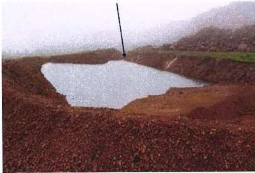
Figure 8: Settling pond near Rayagada dump.
