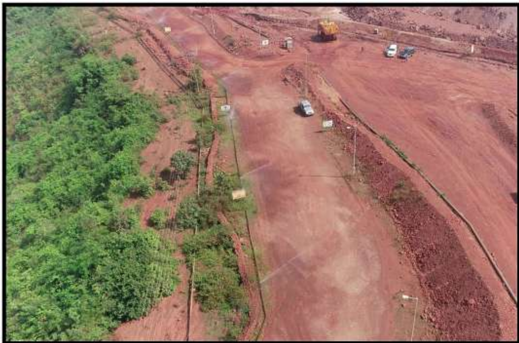
PHOTO 9: Showing Fixed Sprinklers
