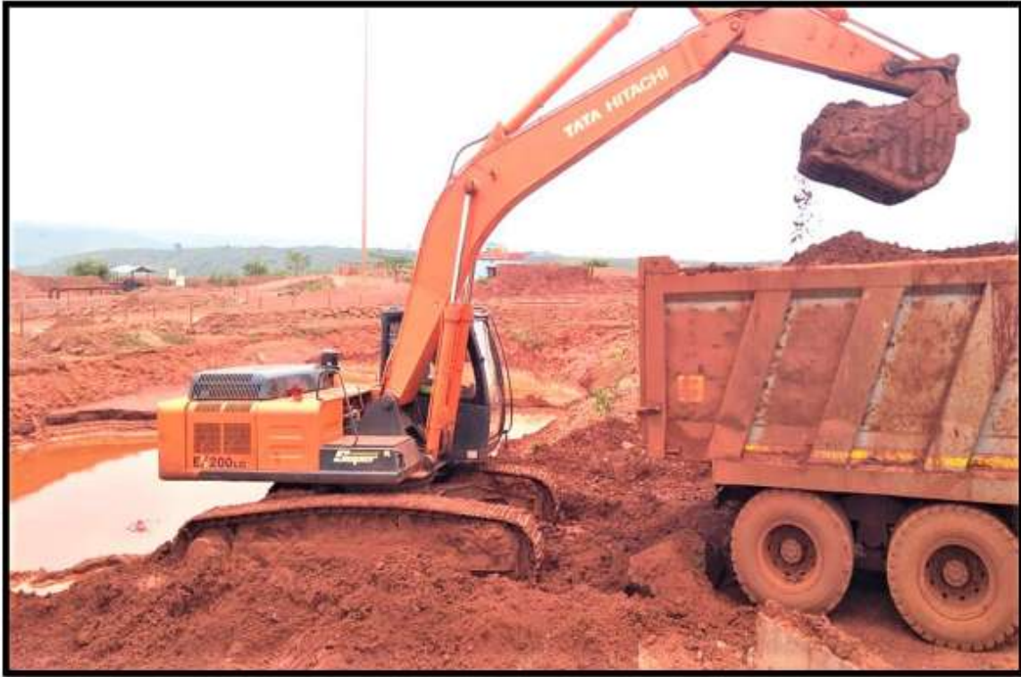
PHOTO 4: Showing Settling Pond Desilting
