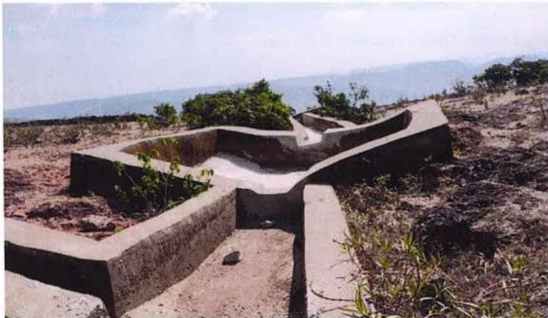
Figure 7: Renovated settling pits
