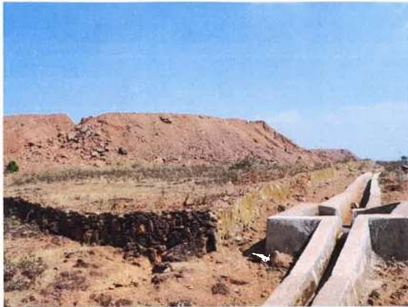
Figure 6: Photographic view of reconstruction of the retaining wall
