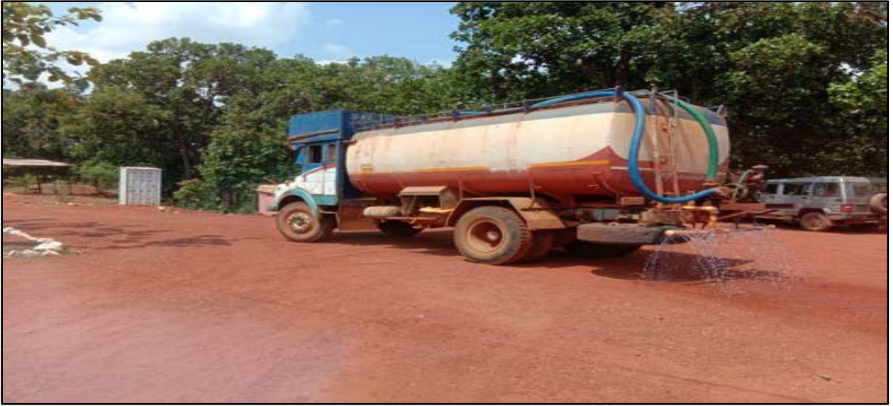
Water Sprinkling for dust suppression
