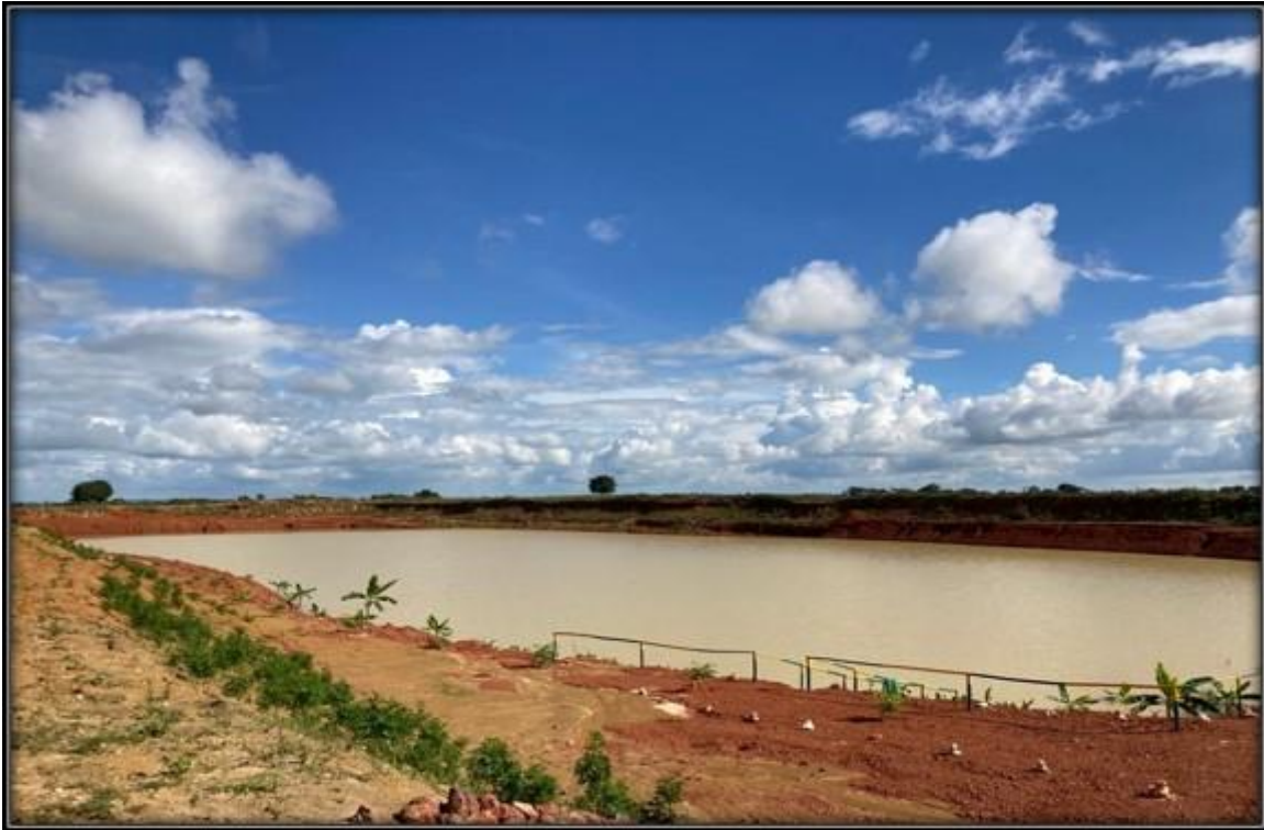
Rain Water Harvesting Pond
