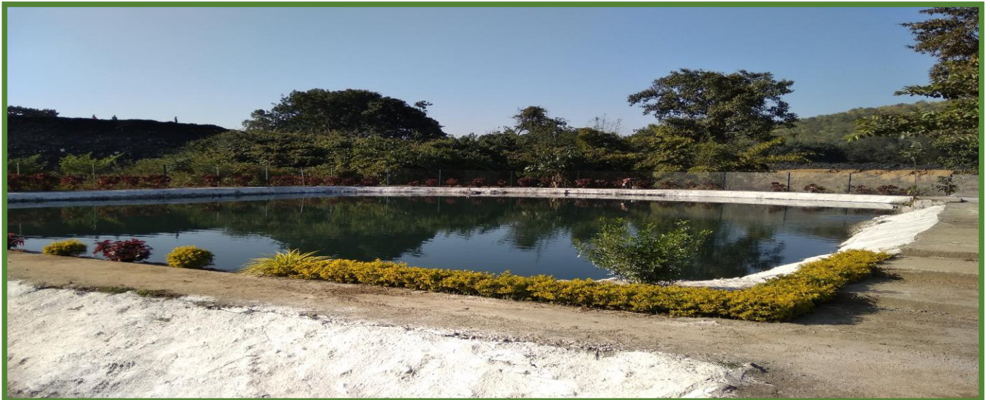
SETTLING POND, NO – 2
