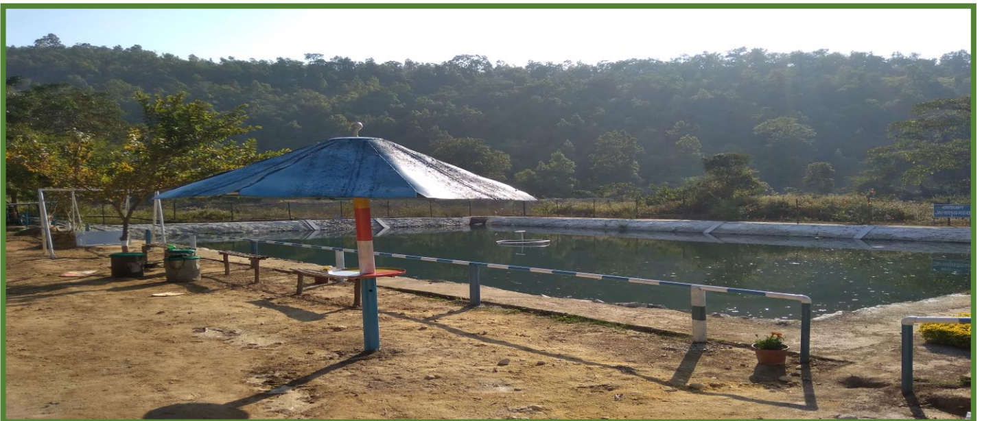
SETTLING POND, NO – 3
