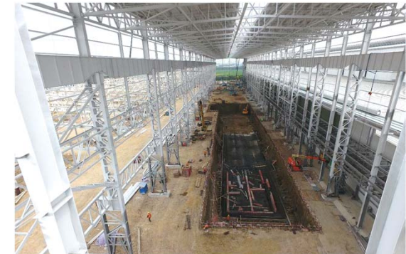
CASH line pit foundation in Changzhou, China
