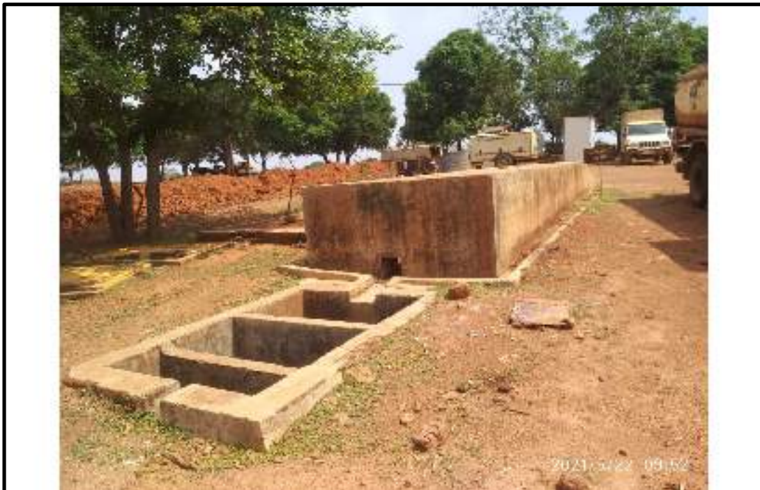
(Washing Ramp and Oil and grease trap)
