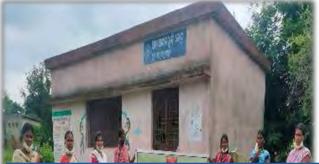
Before Painting at Pandloi AWC
