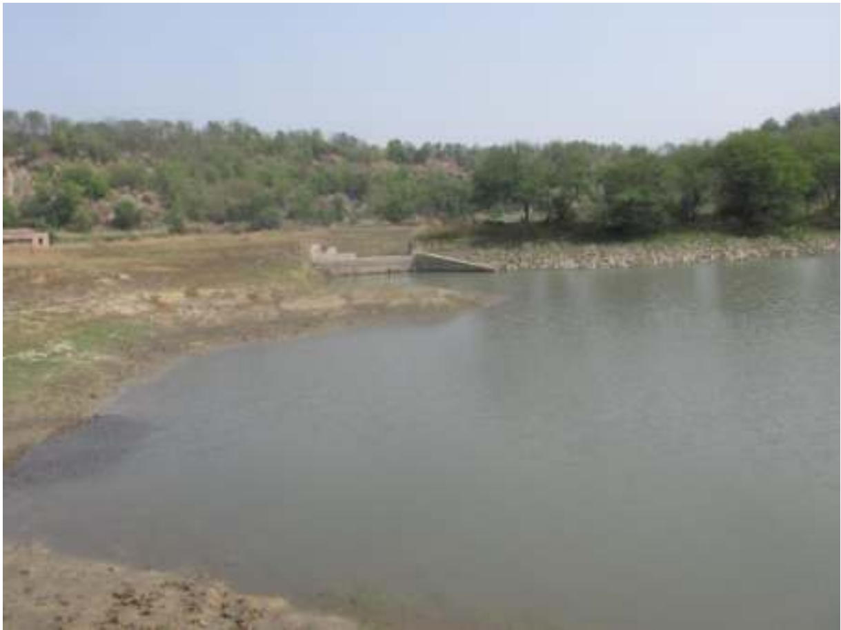
Figure 8: Narayanhara (Water storage and RWH structure)
